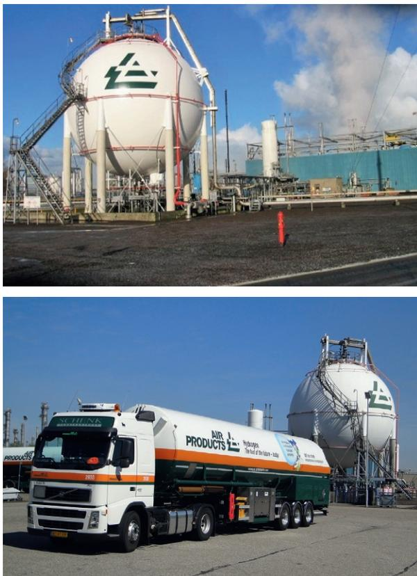
**Figure 2.2** An illustrated overview of a common liquid hydrogen infrastructure: liquefaction in a central plant and storage in a large vacuum-insulated vessel acting as a buffer (top, courtesy of Air Products) and distribution from the plant to the end users by a cryogenic truck trailer (bottom, courtesy of Air Products).
