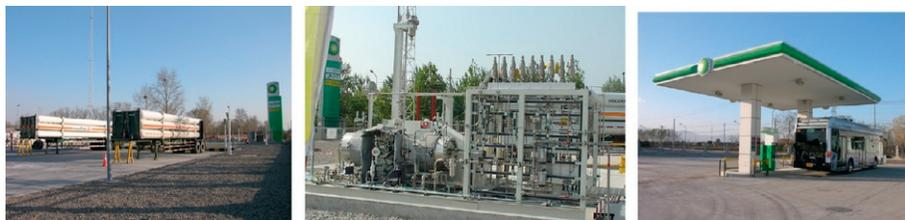
**Figure 13.2** Hydrogen trailers, natural gas reformer, and refueling pump (from left to right) at the Beijing hydrogen park
