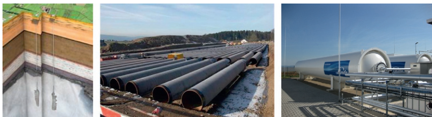
Figure 7.1 Storage concepts for large-scale compressed hydrogen.
